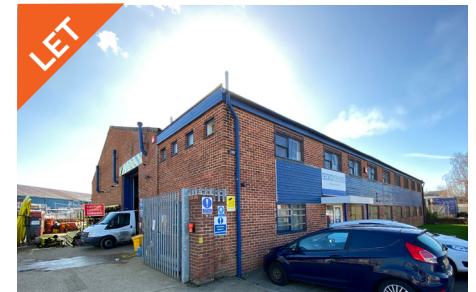
Plot 40, Quartremaine Road Industrial Estate, Portsmouth
