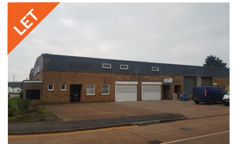
P2 & P2A, Riverside Industrial Estate, Littlehampton
