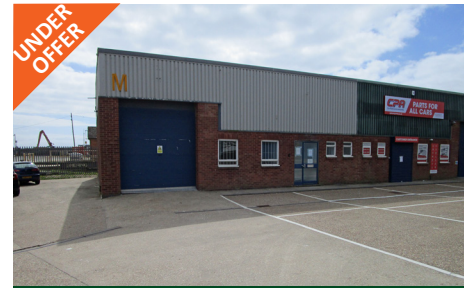
Unit M1, Riverside Industrial Estate, Littlehampton
