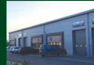
Units 9 – 12, Chichester Business Park From 3,060 sq ft (Total 12,460 sq ft) Let to a private company
