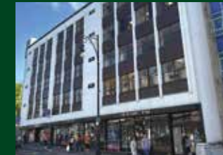
Queens Road, Brighton Office Rent Review on behalf of the tenant
