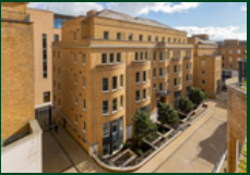
Lanchester House, Trafalgar Place, Brighton 5,167 sq ft Occupier: Avalara
