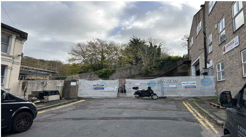
EXISTING VIEW INTO COURTYARD LOOKING EAST
